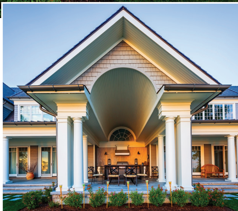
Oversized columns define the covered porch that spans the waterfront façade. A range of sitting areas include an outdoor dining room and kitchen.
